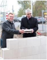
From left to right: Aucotec Executive Officer Uwe Vogt together with Chief Execution Officer and Aucotec founder Horst Beran at the laying of the foundation stone for Aucotec's new head office
